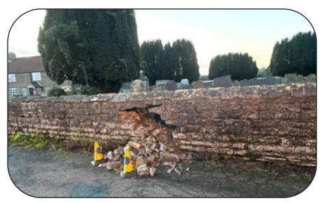
The churchyard wall at St Peter's Claypole has over time seen several types of repair. Last year a section collapsed and repairs began. The winter frosts which could damage the mortar brought work to a holt. There are plans to rebuild it over the coming months.
